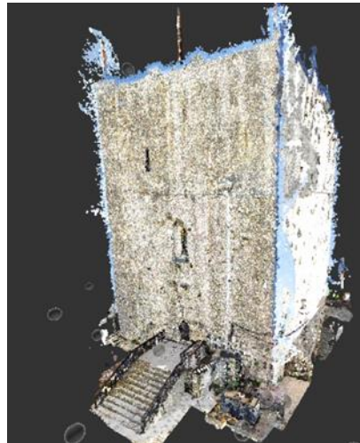
Figure 9. 3D laser scanning of the Tower.
